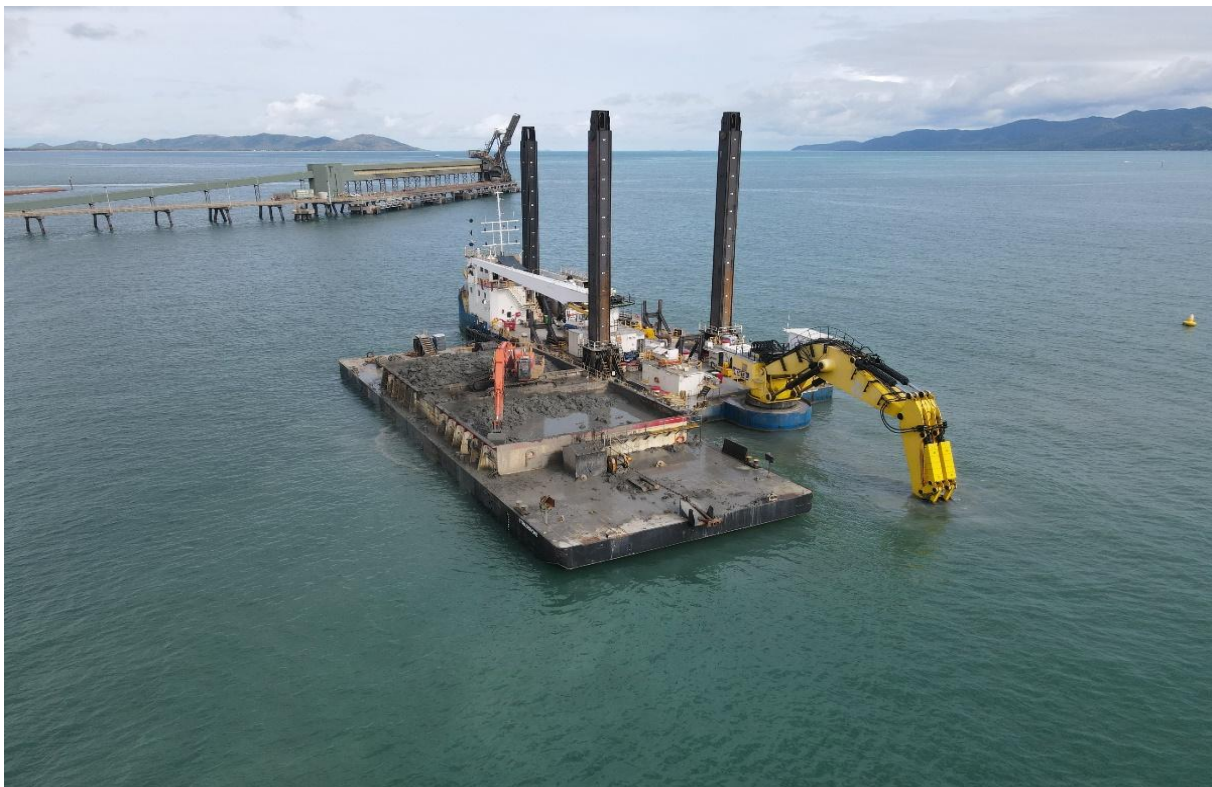
Figure 3: Woomera dredging an approach path to the TUF 2 February 2022
