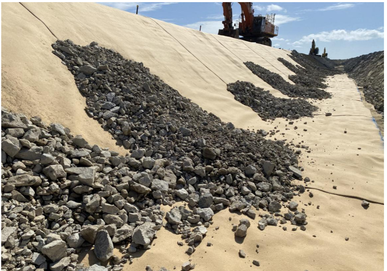
Figure 10: Geofabric is placed along the rock wall as Rear Scour protection works continue August 2024.
