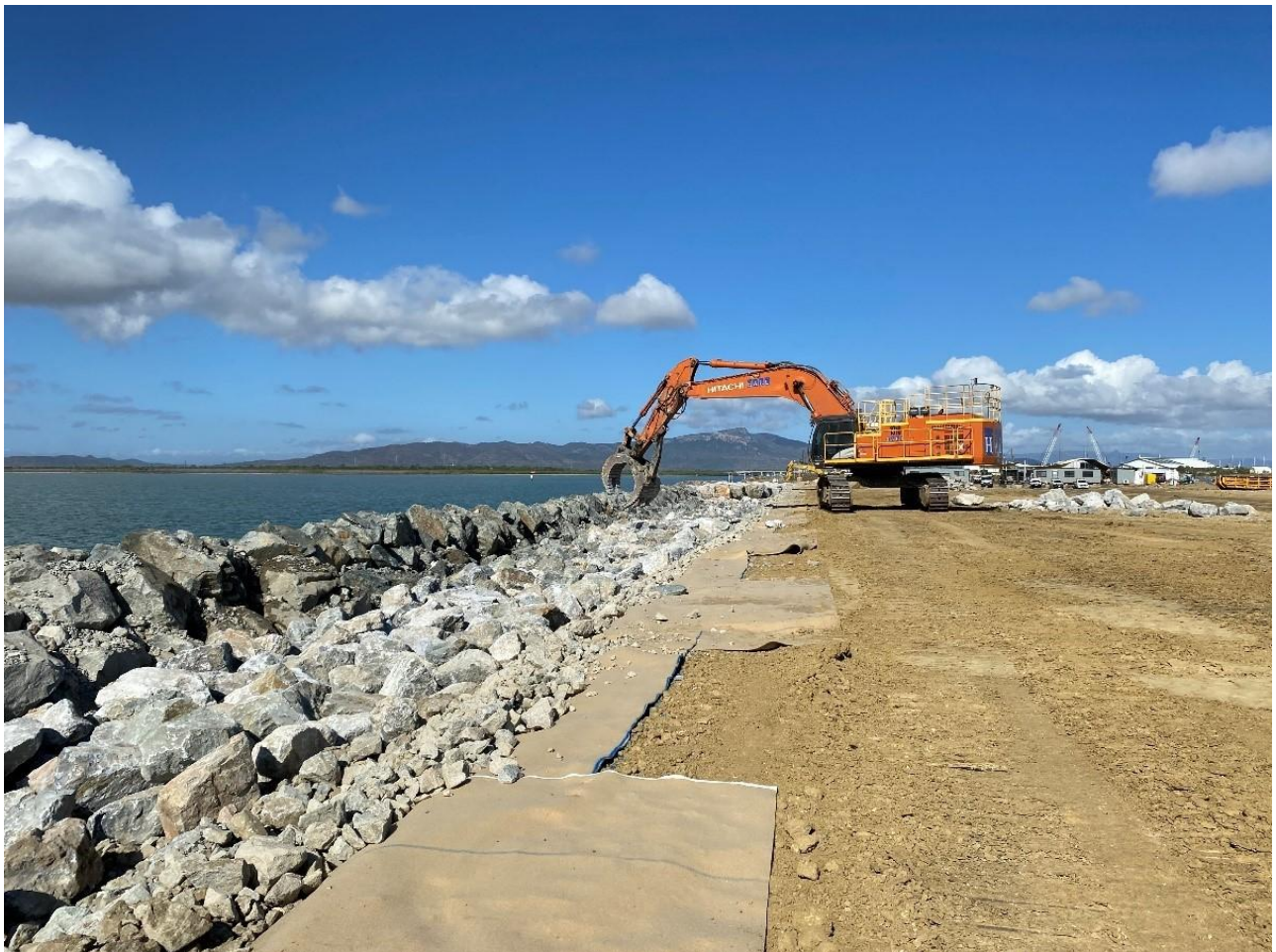
Figure 8: Rear Scour Protection works July 2024.
