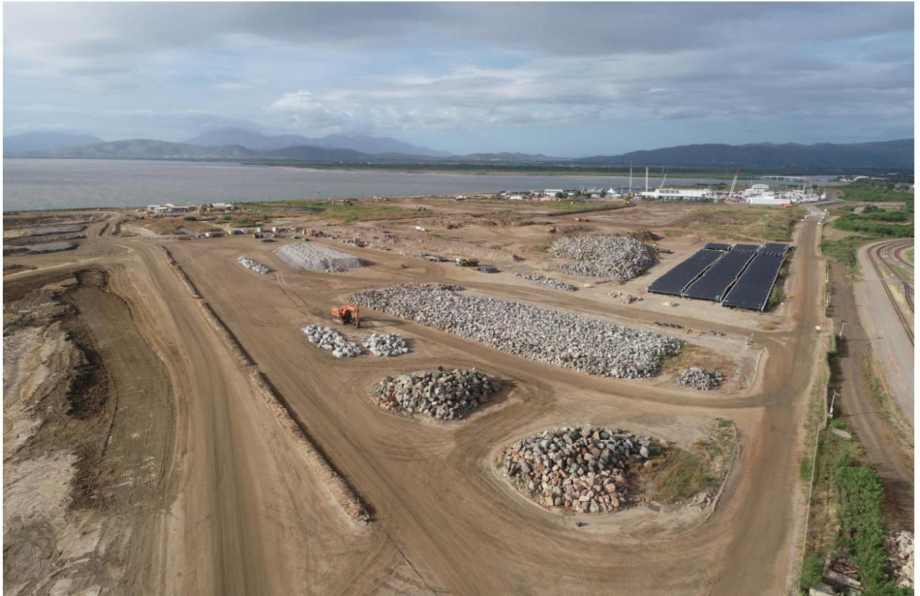
Figure 7: Rock stockpile for Rear Scour Protection May 2024.
