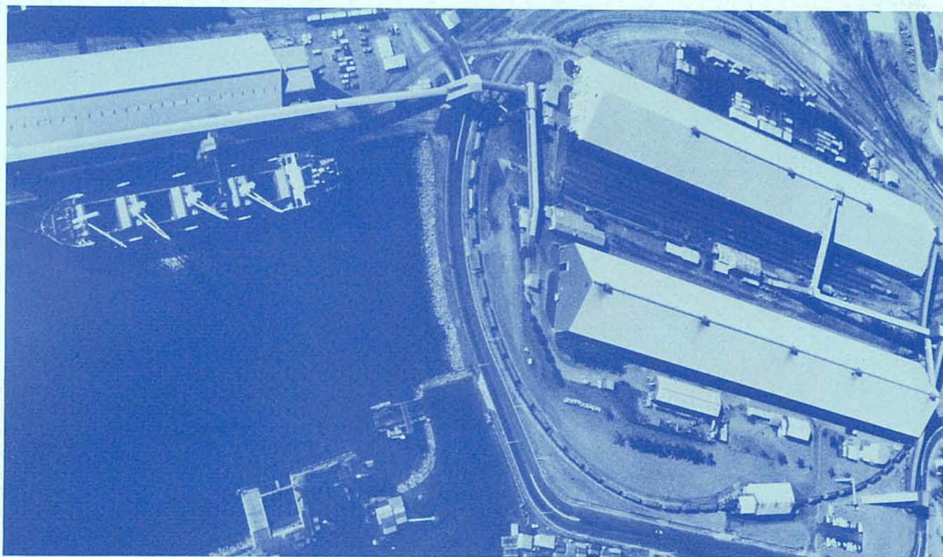
Sugar handling at Townsville is fully automated with the completion of the rail loop.
