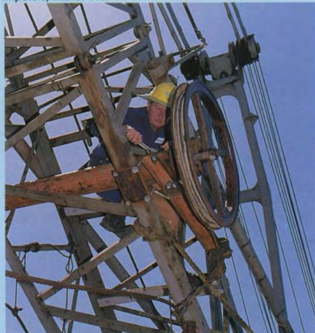
TPA employee Mr. H. Thorley repairing dredging plant.
