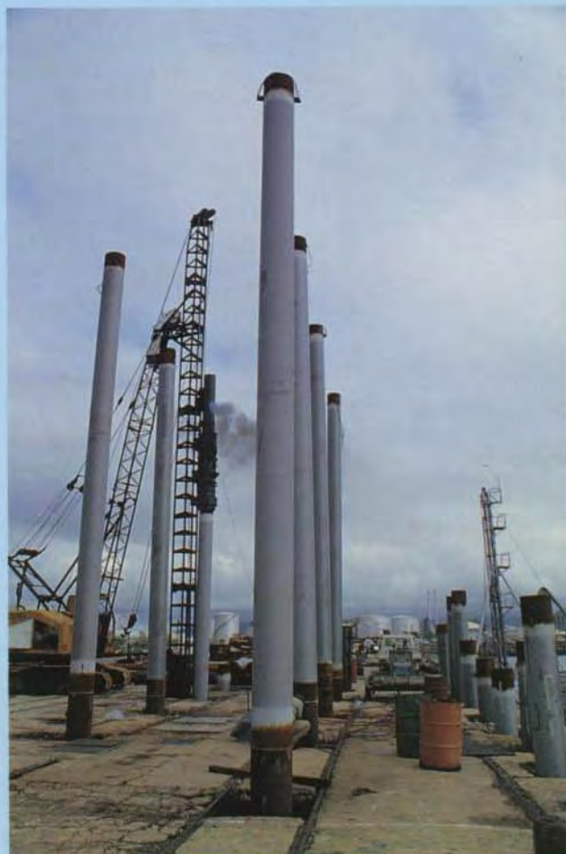
Driving piles during reconstruction of No. 4 Berth for import of Nickel Ore.
