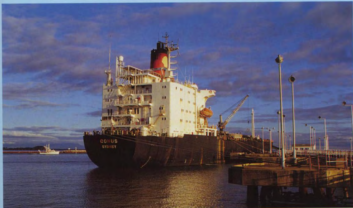
M.T. Conus discharging petroleum products at No. 1 Berth.
