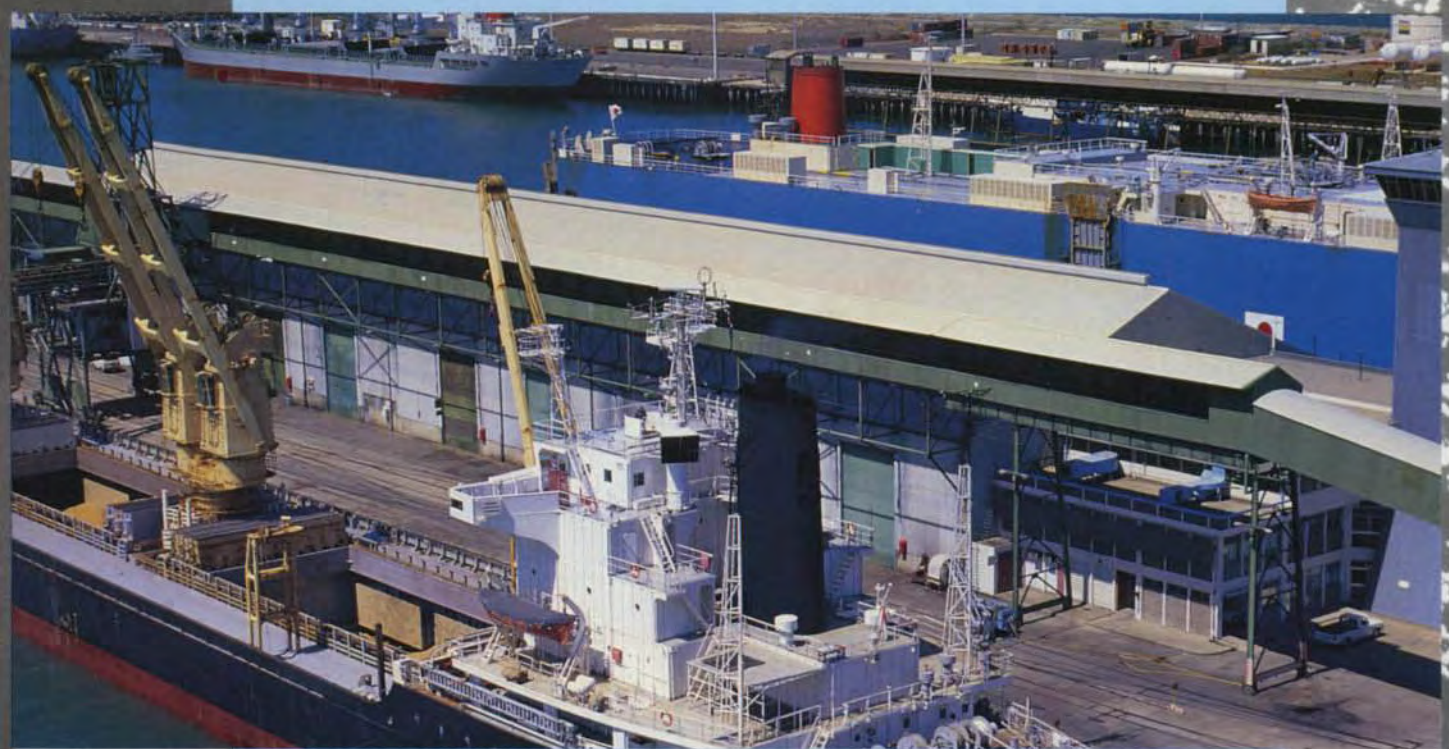
Loading sugar at No. 9 Berth (foreground) — Unloading motor vehicles at No. 8 Berth (middle) — Loading Mt. Isa metals at No. 2 Berth (background).
