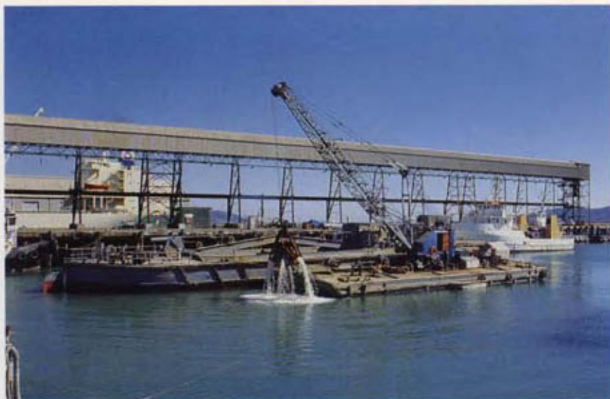
Above: The Authority's grab dredge in operation at No. 4 berth. The mud spoil is loaded on to a mud barge. No. 4 berth is presently used for bulk liquid cargoes and light general cargo.
