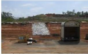
Above: Black plastic stormwater chutes installed at Warren's Hill Waste Management Facility.
