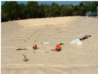
Above: Replacing floating roof at Depot Water Treatment Plant.
