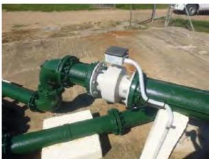
150mm flow meter monitoring water transfer from the low lift to high lift
