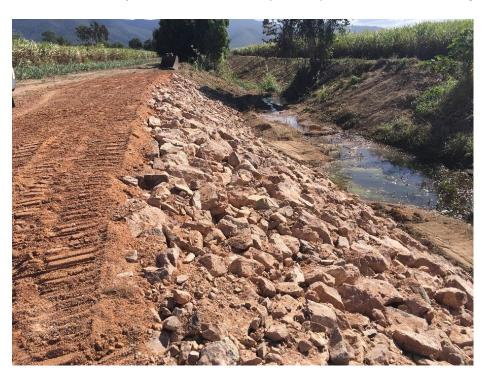
Herbert River (HR-2). Works to commence about 7/9/2020. After access to riverbed was completed, about 40% of the rock and fill are now in place for the bench, rock protection and top of bank earthworks.
