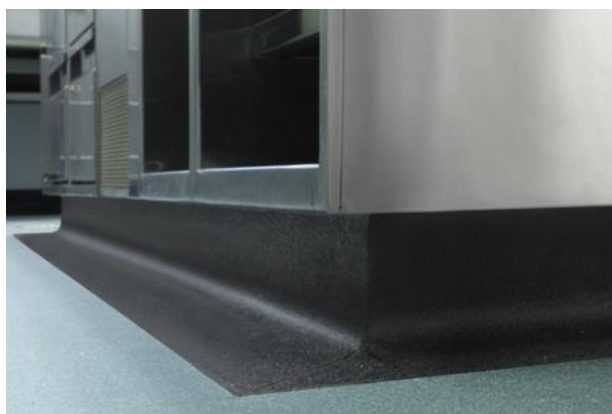
Figure 2: Example of a plinth with coving
