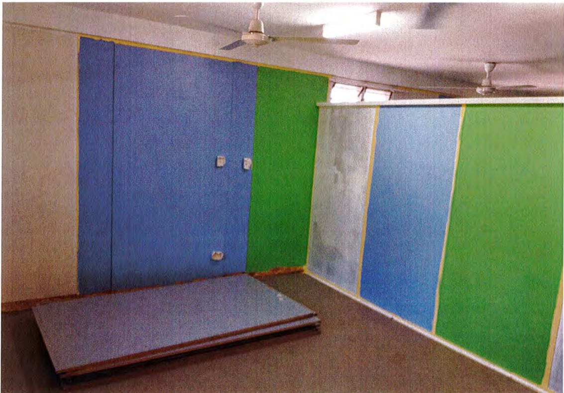
Consolidation Of Boarding Renovations In Works
