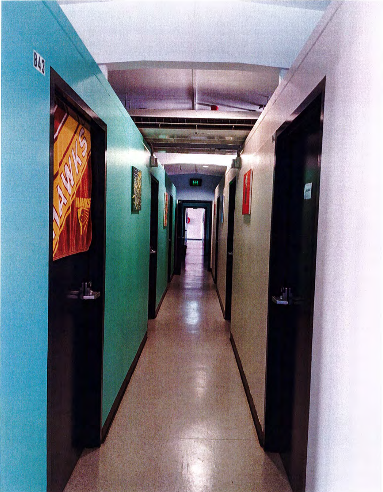
Consolidation Of Boarding Renovations In Works
