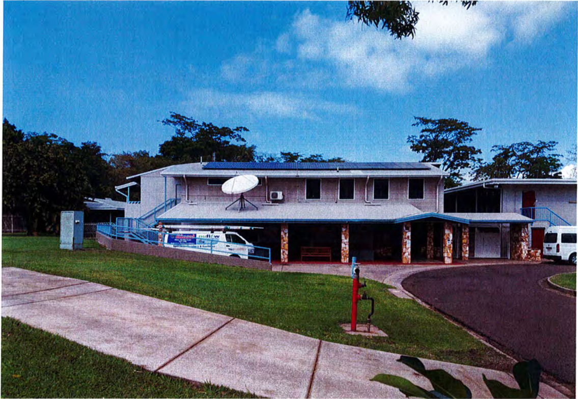
Consolidation Of Boarding Renovations In Works
